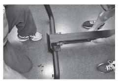
**6.** Attach the front curved tubular floor brace to the post. Using four hex head bolts 3/8" x 5/8" long bolts, screw down until firmly tight.
